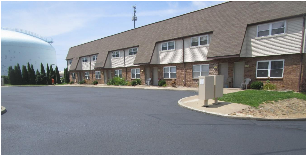
Photo of Walnut Woods Community. Photo credit to Bloomington Housing Authority.
